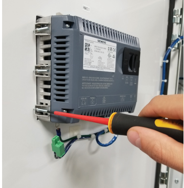
Figure 3 Loosening HMI fasteners.
