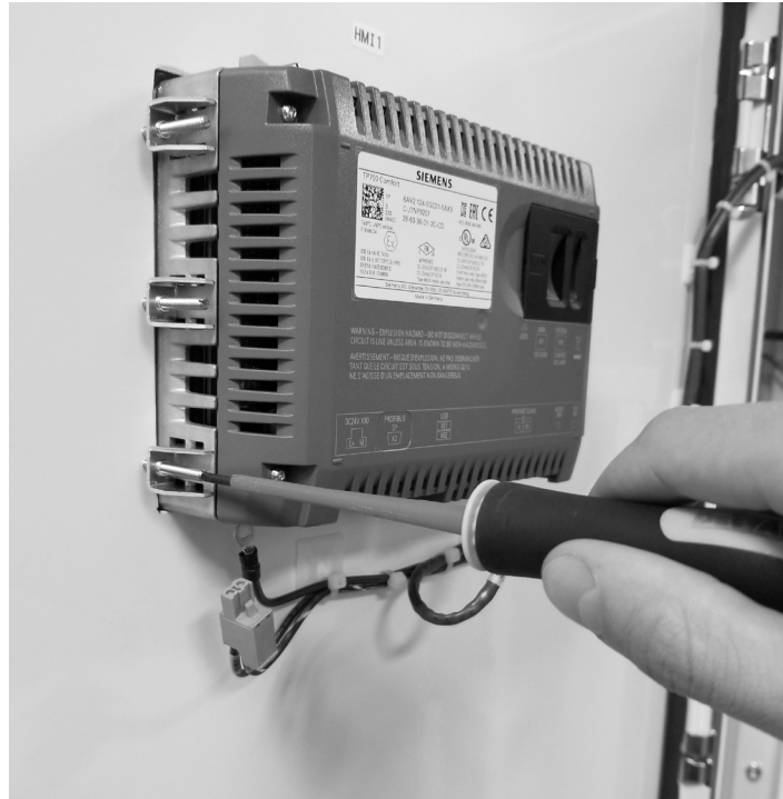
Figure 2.3.3 Loosening HMI fasteners.
