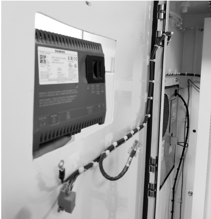
Figure 2.3.5a Removal of the HMI from the front of the enclosure.
