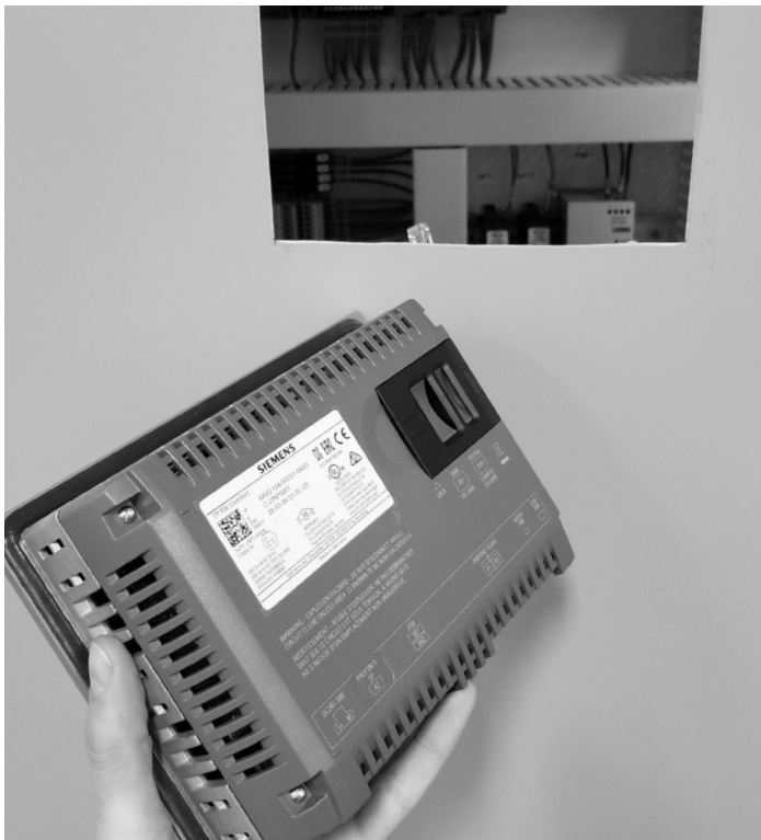
Figure 2.3.5b HMI completely removed.
