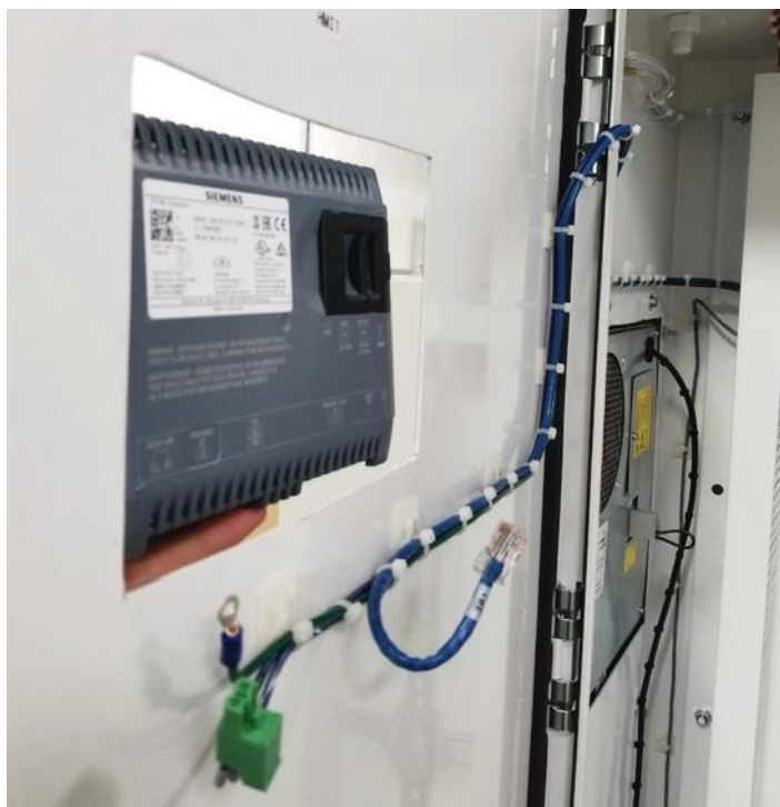
Figure 5 Removal of the HMI from the front of the enclosure
